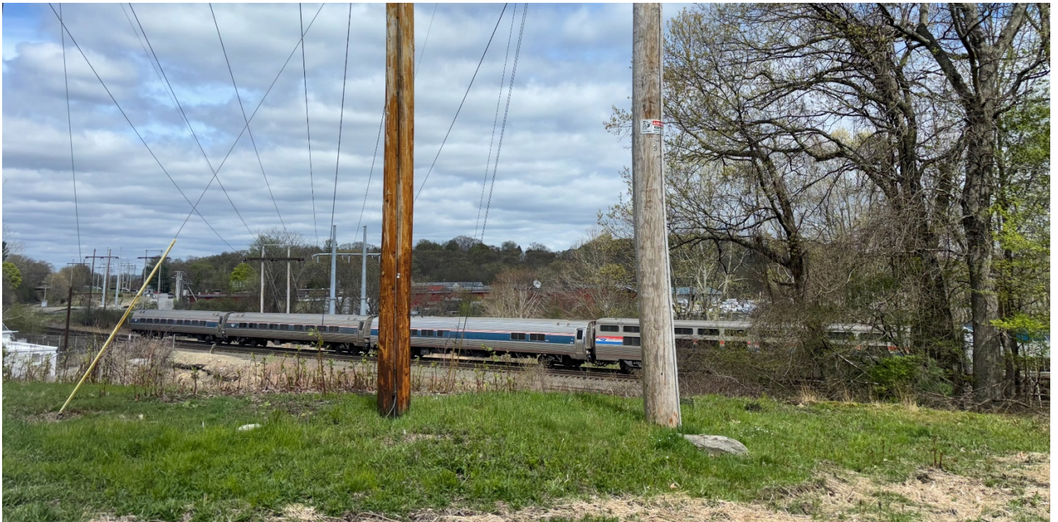
Photo #6: Pole 9 (Tap 2 #9) on the WS2 Line, located within BLSF. Facing northeast
