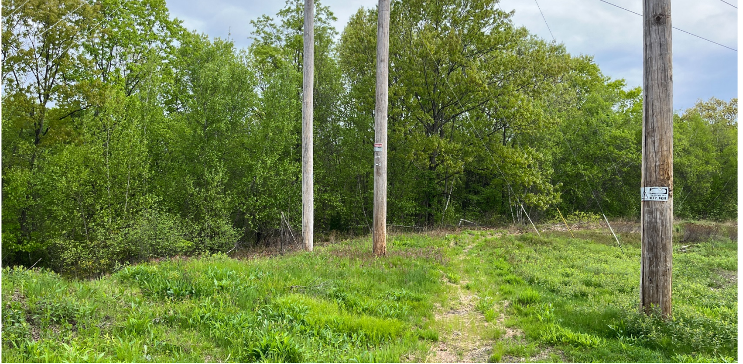
Photo #5: View of Pole 22 on the WS1 Line, located within the 100-ft Buffer Zone to BVW. Facing North
