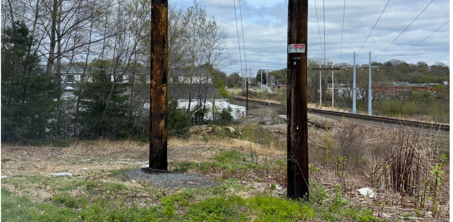
Photo #1: View of Pole 9 (A127E #10) on the WS1 Line, located within the Bordering Lands Subject to Flooding (BLSF). Facing East
